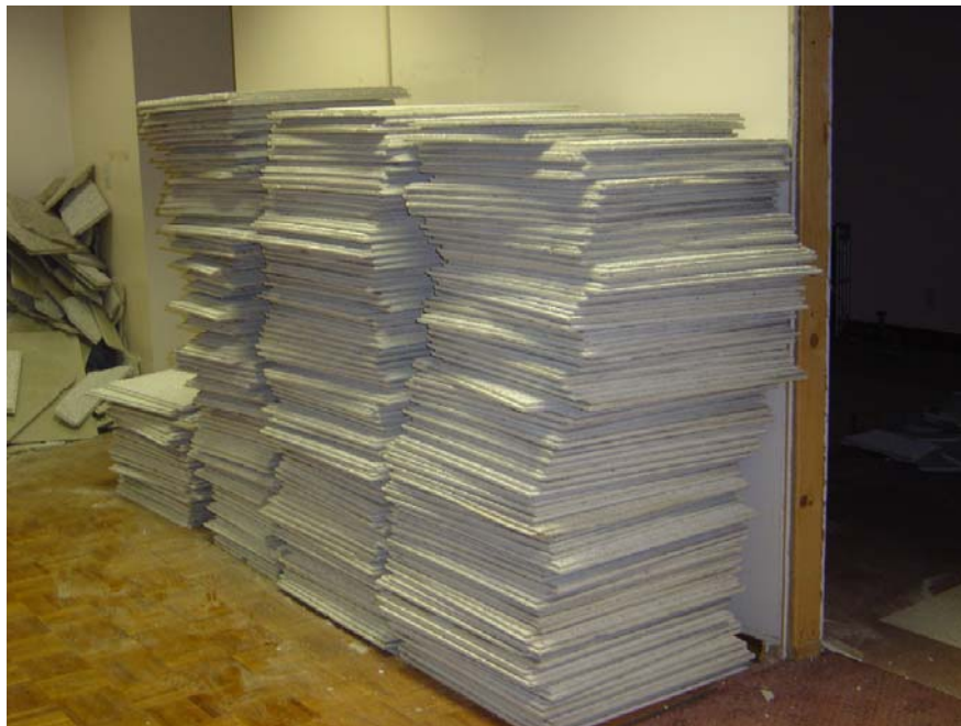
Photo 6. Salvaged ceiling tiles from 132 W 32 nd Street. The broken tiles were picked up by Armstrong for recycling.
