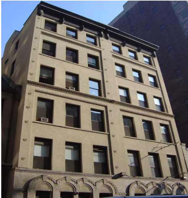
Photo 1. Front Elevation of the 6-Story Building at 134 W 32 nd St.
