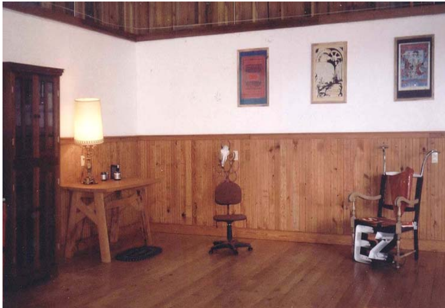
Figure 2. Reuse Education Center at Beyond Waste, Cotati, CA demonstrating value-added reclaimed wood products such as wainscoting, flooring, and furniture.
