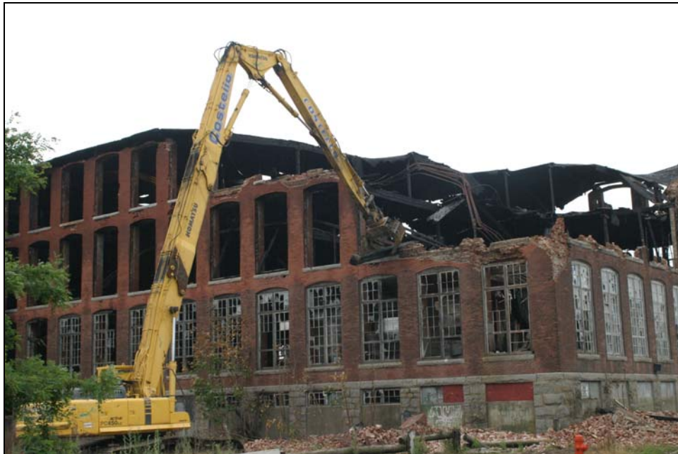
Figure 1: Dismantling a New England Mill Building
