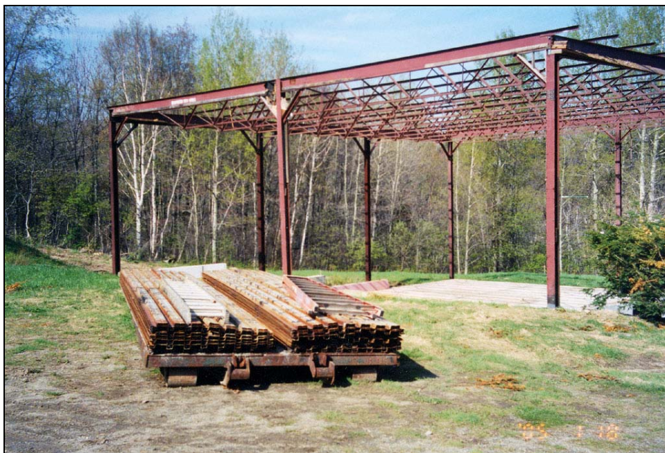
Figure 3: Dismantling of Steel-Framed Building for Reuse
